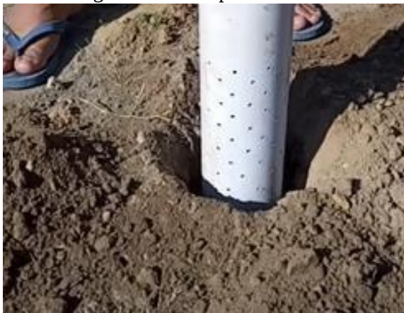
Figure 3. Inserting PVC Pipe into Pre-perforated Soil
