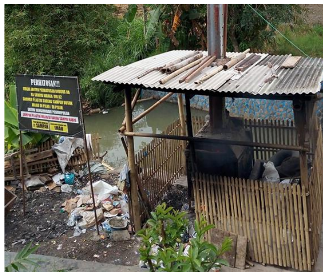
Figure 1. Condition of the Waste Disposal Site in Sukawening Village (Source: Author's Documentation)
